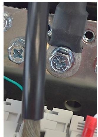
Figure 9 Connecting the battery
